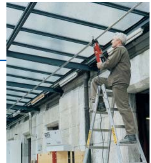
Fire extinguishing systems
